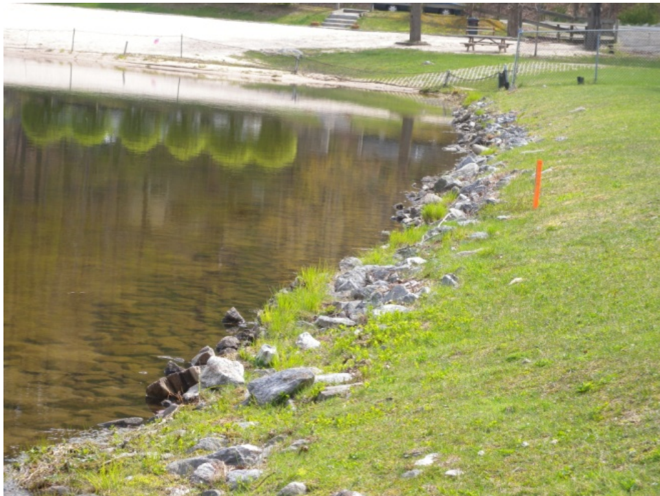
Photo 2 - EOH-07 Upstream Slope
