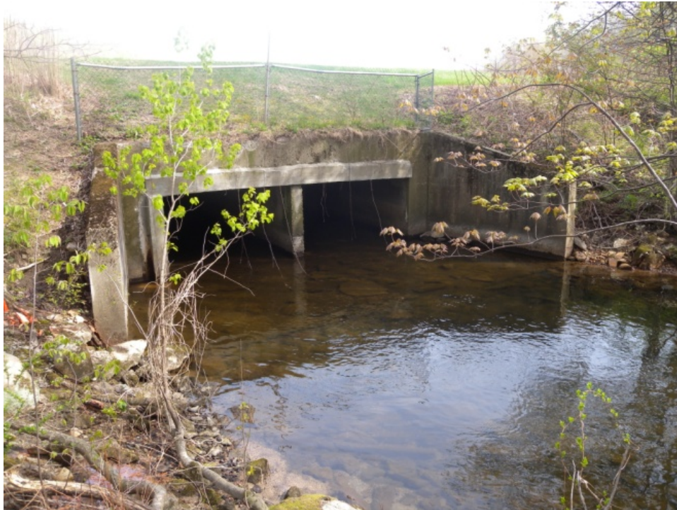
Photo 9 - EOH-07 Spillway Discharge Outlet
