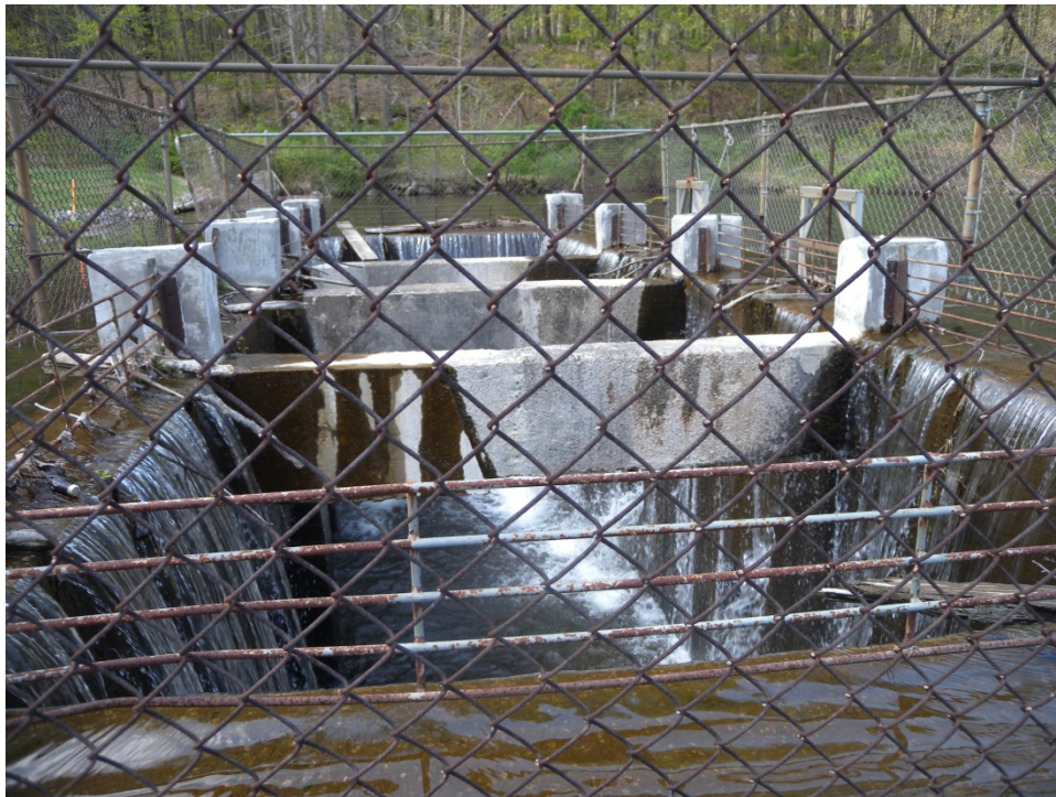
Photo 8 - EOH-07 Drop Inlet Spillway
