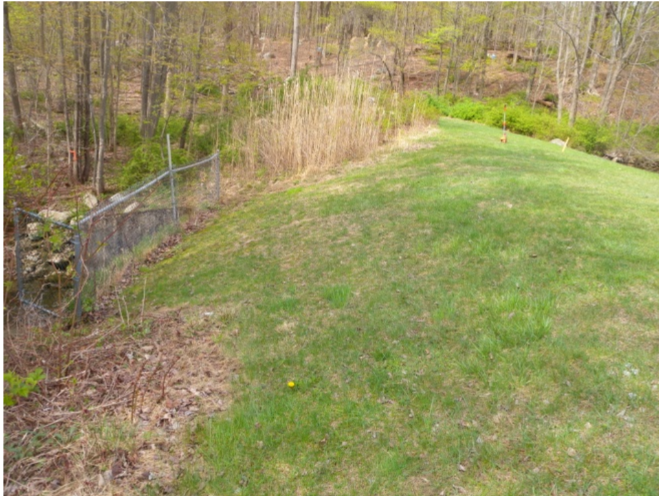
Photo 3 - EOH-07 Downstream Slope
