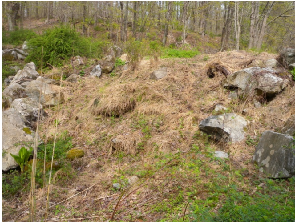
Photo 5 - EOH-07 Right Abutment Downstream Slope
